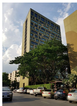
Promphan building 3 7th Floor
